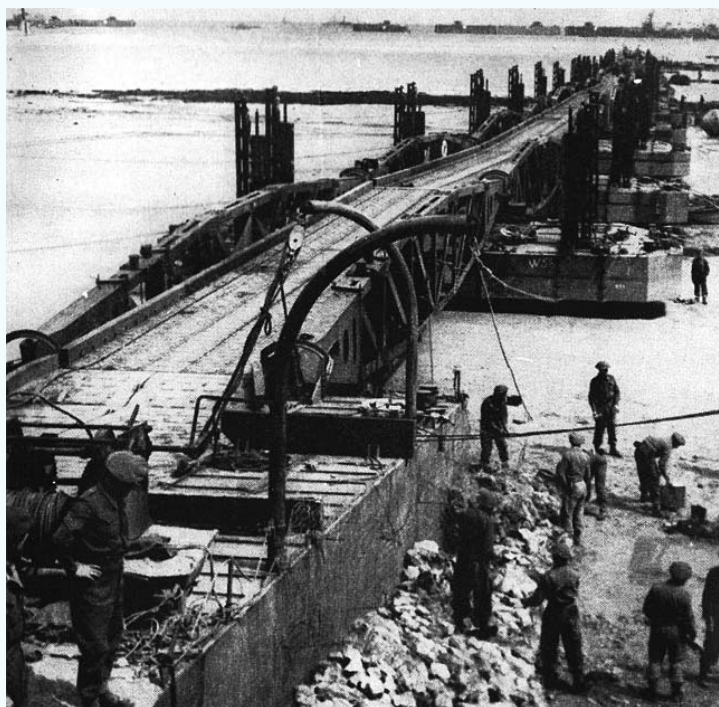
(above) 'Beetles' and roadway units. The 'Beetles' were the pontoons which supported the roadways. There were two types of 25m (80ft) roadway units - Class 25 and Class 40, capable of carrying 25 and 40 ton loads respectively. In the foreground, is a shore ramp.
