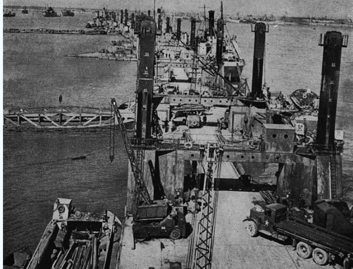
'Spuds'. The 'Spuds' were arranged in a row, roughly parallel to the shore, linked by bridge units and buffer pontoons. The roadways can seen, heading to the shore.
