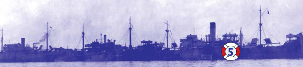
'Phoenix'. The concrete caissons did not have a continuous deck. Anti-aircraft guns were mounted on towers on many of the 'Phoenix'.
